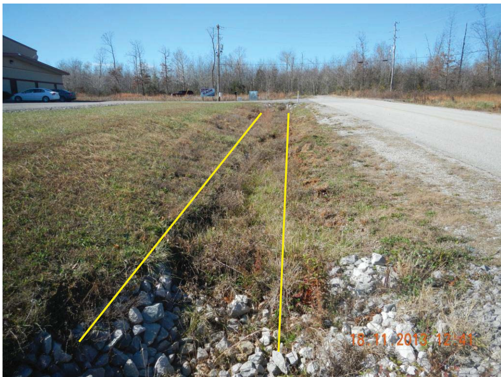
Photograph 4 – DSCN 1861. N35.3976°, W-86.1214°. View of WWC-1 facing up gradient and west toward PND -1 outfall point.
