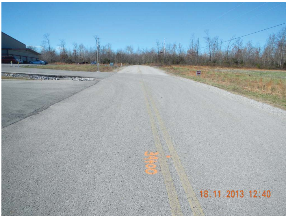
Photograph 2 – DSCN1855. N35.3976°, W-86.1209°. View of the proposed alignment facing west at Murray Drive.
